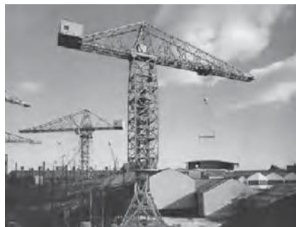
Cranes at Work
