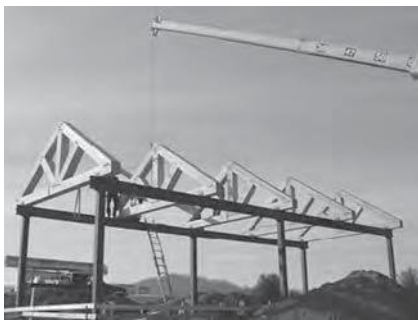
A Timber Frame Truss
