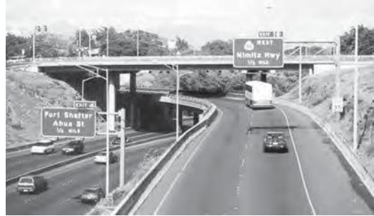
Flyovers and Highways in Hawaii
