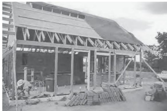
A structure showing a horizontal beam in front
