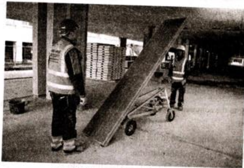
Fig. 1.1 Wagons used in precast unit
