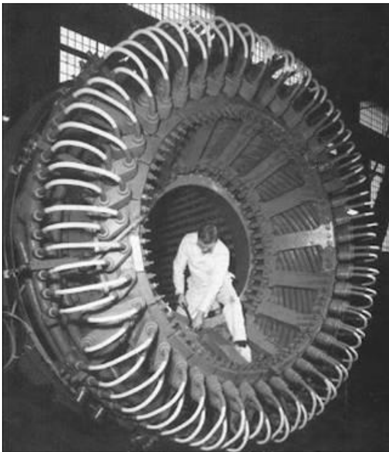
Fig 3. (a) Stator of a salient pole alternator
